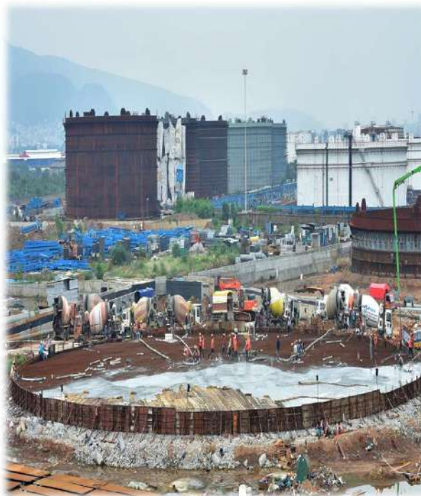
TANKAGES (51 ACERS) 66 DIA MTR Tank pad - 30000 Cum– PROJECT – VISAKHAPATNAM - ANDHRAPRADESH
