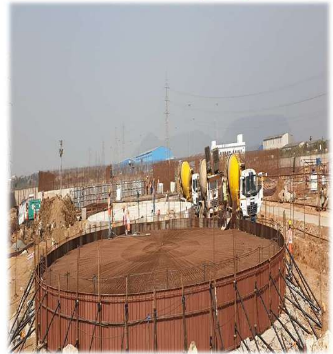
SBR FEED TANK PAD - IETP - HPCL – VRMP VISAKHAPATNAM – ANDHRAPRADESH - INDIA
